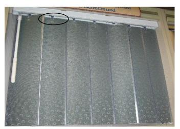
3. Rotate the louvers open. Slide a hard plastic card between the louver and the long side of the louver stem. Push the card and louver up toward the top of the louver stem. This will unseat the louver from the louver stem.
