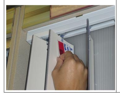
4. Remove the louver by pulling down on both the louver and plastic card at the same time. Lay louver on a clean flat surface. Repeat for all louvers.
